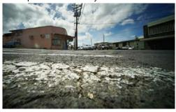
This type of cracking in Kalihi can cause potholes if enough water gets under the pavement.
