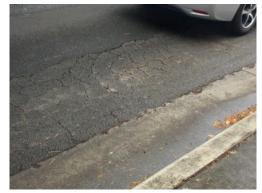
"Alligator" or "crocodile cracking" on Punchbowl Street. When the cracks are sealed, the treatment looks like winding, black lines placed over the cracks.
