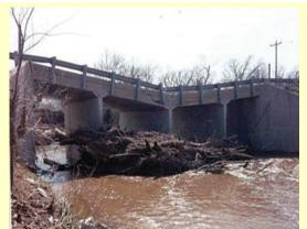
Photo: Oklahoma DOT More than wear and tear, debris accumulation can accelerate a bridge's structural undermining.
