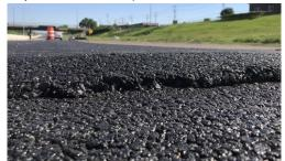
**Concrete Paving Association of Minnesota** The old concrete bubbled up under a new layer of asphalt last month during repair work on Interstate 94 in Minneapolis.
