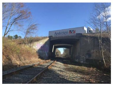
Of the 32 Cumberland County bridges considered structurally deficient, the U.S. Route 1 railroad overpass in Freeport was rated lowest at 4 for its deck and superstructure.
