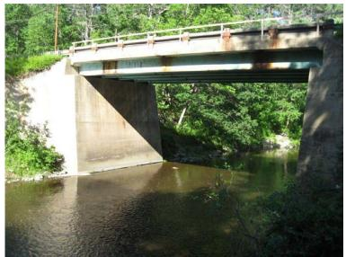
The bridge spanning the Little River between Gorham and Windham on Routes 202 and 4 was considered structurally deficient for its deck and superstructure. It was replaced last summer.
