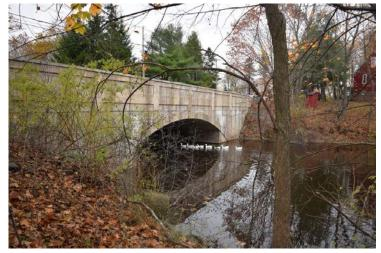
Built in 1989, the deck on the Congress Street bridge over the Stroudwater River in Portland is considered structurally deficient because of its substructure.
