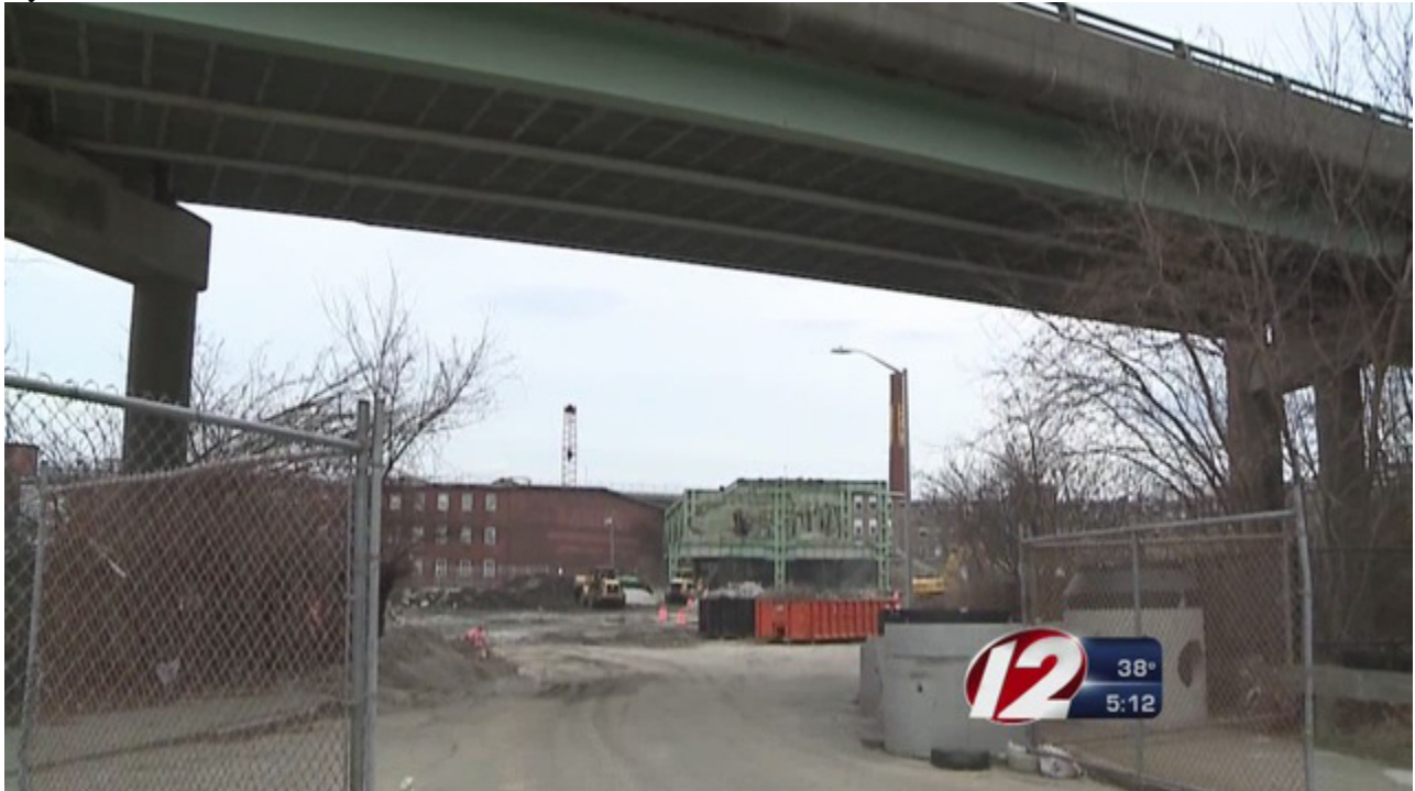
Route 9 construction project in Fall River
