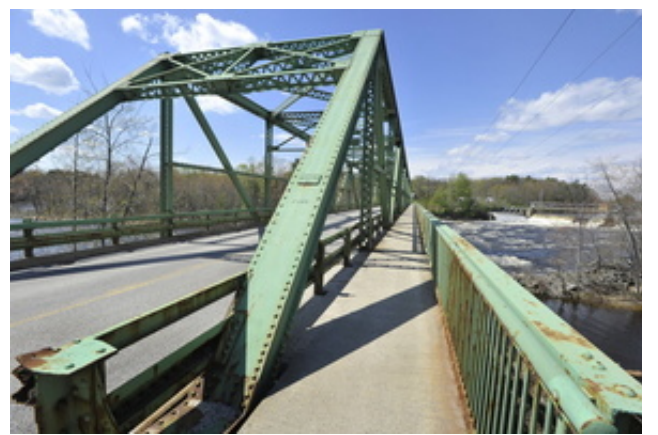
One high-priority project is the Bar Mills Bridge carrying Route 4A over the Saco River at the Buxton-Hollis line.
