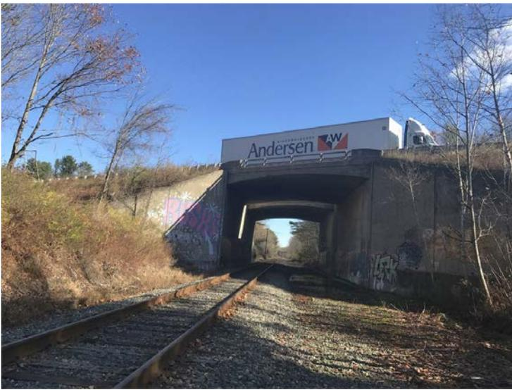
Of the 32 Cumberland County bridges considered structurally deficient, the U.S. Route 1 railroad overpass in Freeport was rated lowest at 4 for its deck and superstructure.
