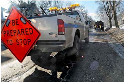
A City of St. Paul Public Works truck diverts traffic around street service workers filling potholes on Smith Avenue Wednesday March 12, 2014. (Pioneer Press: Jean Pieri)
