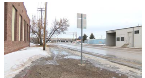
Projects jump started by the loan include adding sidewalks along 14th and 15th streets N, from 8th ave. N to the river.
