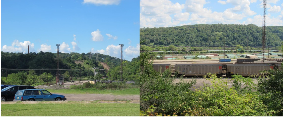
The proposed Mon-Fayette expressway extension would sit atop this hillside in Duquesne (left), cross above Route 837 and provide easy highway access to manufacturing companies and train depots along the Monongahela River (right). Credit Liz Reid / 90.5 WESA
