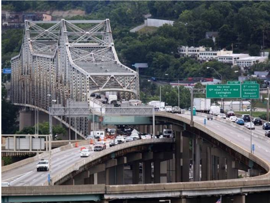
The Brent Spence Bridge is undergoing extensive maintenance. The work means closed lanes, detours, traffic back-ups and headaches for commuters. (Photo: The Enquirer/ Liz Dufour)
