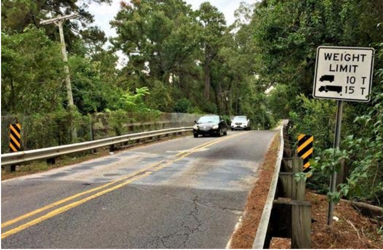
This overpass on Military Highway is one of more than 50 bridges in Rapides Parish that is structurally deficient.
