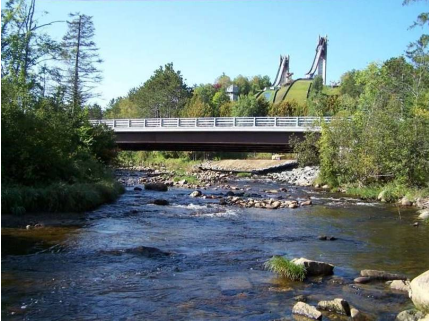
More bridge and road work is needed in New York, where 52 percent of the bridges are 50 years old or older, according to TRIP's new report. The organization would like to see more projects like the bridge on Route 73 south of Lake Placid, shown above, that was completed in 2017. Photo by NYSDOT
