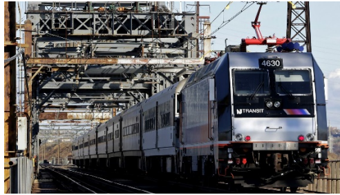
A New Jersey Transit train travels across Portal Bridge in Kearny, N.J., in 2014. Plans call for a pair of replacement bridges for the 105-year-old structure. (Julio Cortez / Associated Press)
