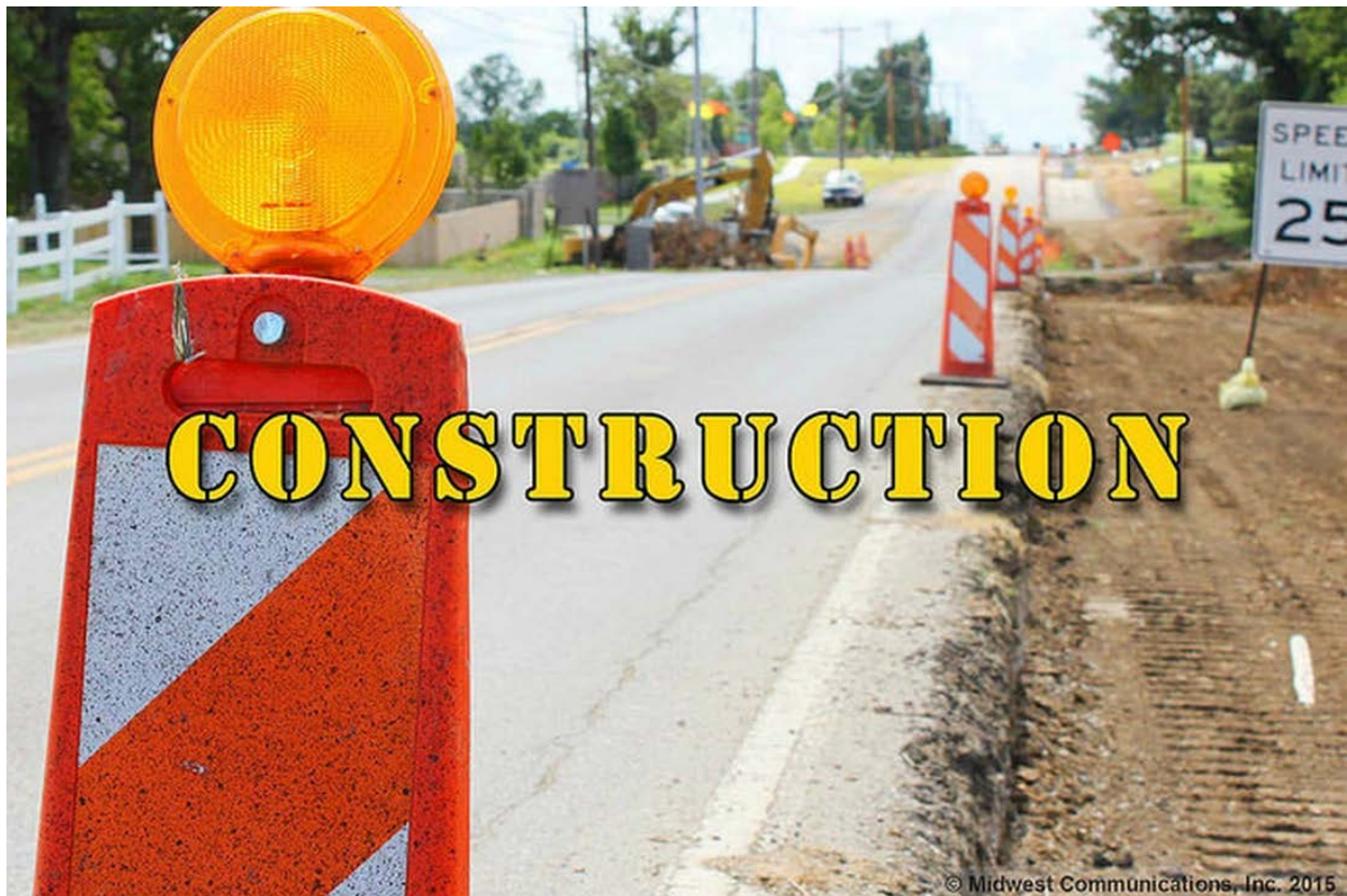
Road Construction (image © Midwest Communications)
