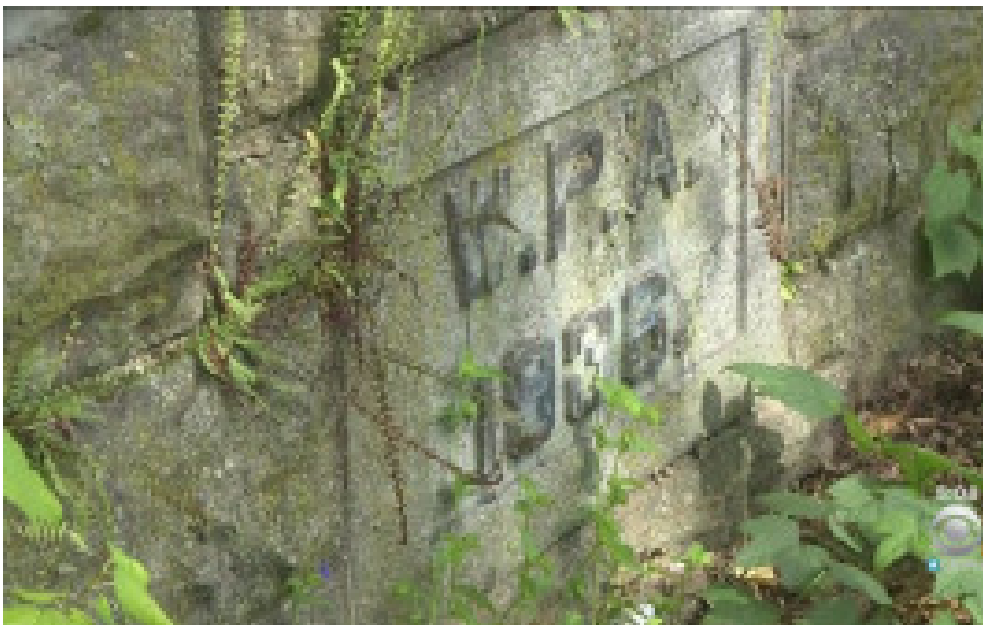
Hillside Avenue Bridge in Mamaroneck. (Photo: CBS2)
