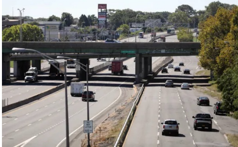
A view southbound of Central Park Avenue, right, and I-87, left in Yonkers Sept. 17, 2019. The Cross County Parkway that crosses over both roadways, is pictured above. (Photo: Mark Vergari/The Journal News)
