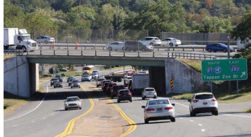
This is view of bridge of I-87 over Route 303 in Nyack Sept. 17, 2019. Thirteen percent of bridges in the Hudson Valley are rated in poor/structurally deficient condition, according to a new report released today by TRIP, a Washington, DC based national transportation research nonprofit. (Photo: Carucha L. Meuse/The Journal News)
