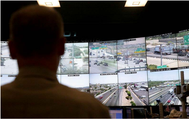
A worker monitors some of the hundreds of surveillance cameras that the Arizona Department of Transportation has installed in Phoenix and Tucson, allowing it to respond quickly to problems. A new report says Arizona had the highest rate of fatalities on its interstate highways in 2018. (Jessica Alvarado Gamez/Cronkite News)
