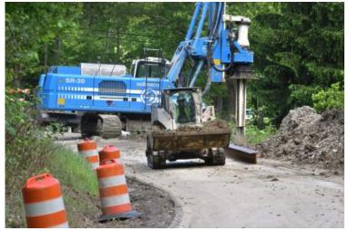
Photo by Scott McCloskey Crews with the Ohio-West Virginia Excavating Company make slip repairs and construct a new retaining wall on Peters Run Road in 2019. Poor road conditions cost drivers in the Wheeling area \$1,421 annually, according to TRIP.
