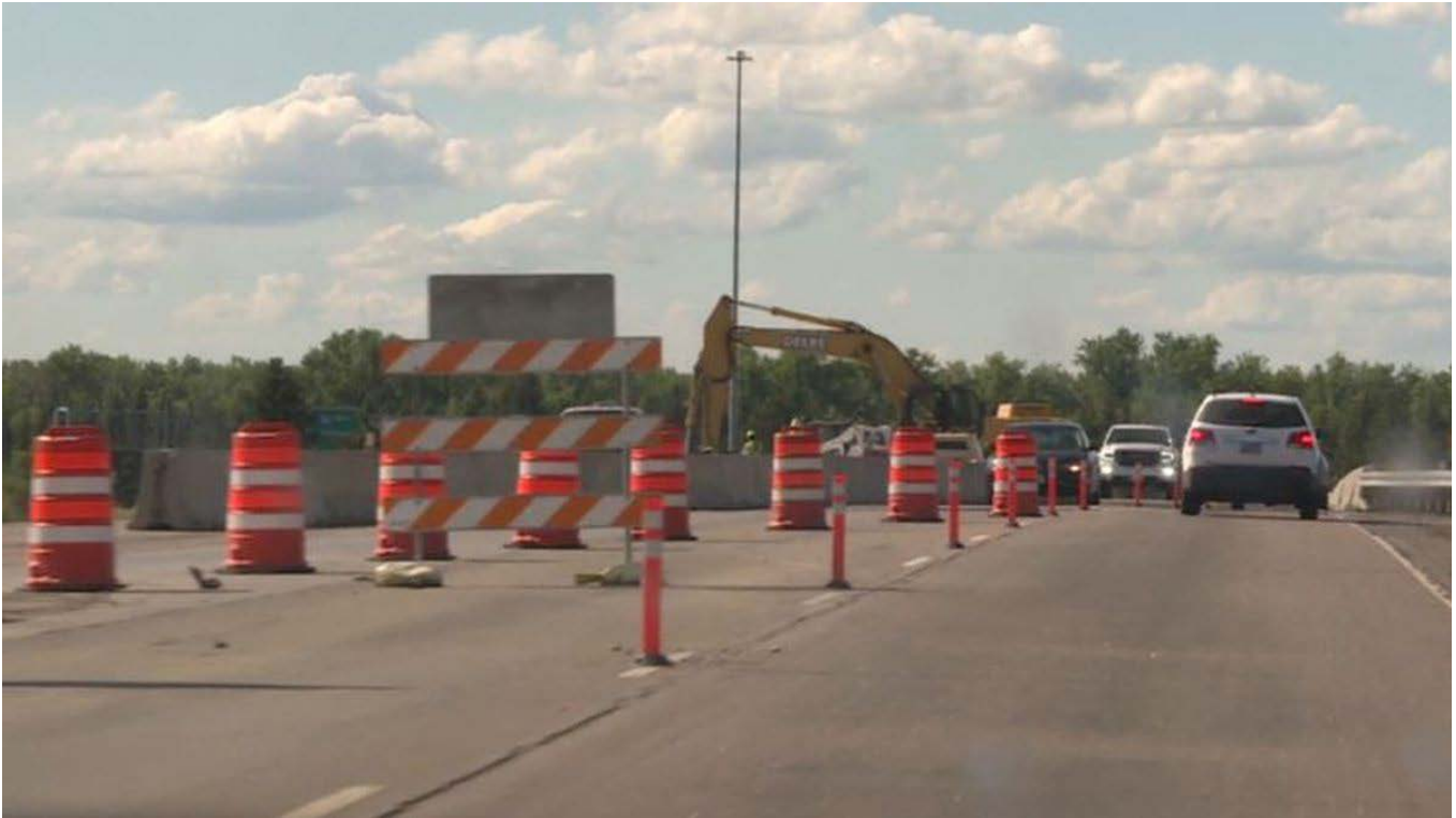
North Dakota Road Construction (KFYR)
