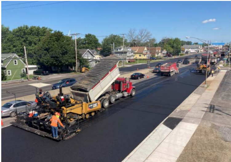
Road repaving. NYS Department of Transportation photo.
