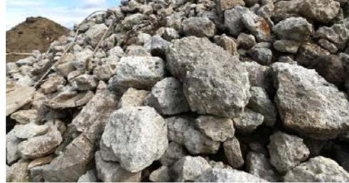
Chunks of the former I-275 concrete highway are piled up, Thursday, April 7, 2022, before being transported to the concrete-crushing plant to be crushed, treated and tested then reused as the new I-275 aggregate base. The Revive 275 Project is a 14-mile, four-year-rebuild project. *Todd McInturf, The Detroit News*
