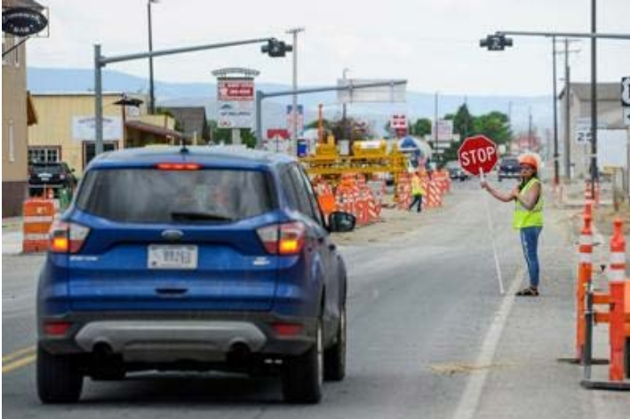
A construction flagger halts traffic on U.S. Highway 12 in Townsend in 2021 as crews work on a road upgrade project. THOM BRIDGE, Independent Record
