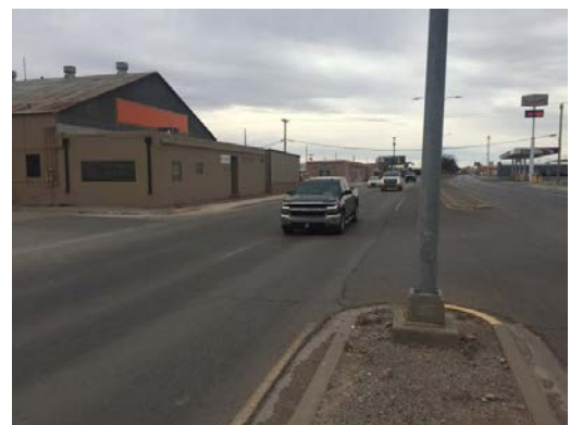
Traffic heads north along U.S. 285 in Artesia on Feb. 21, 2023. A recent study indicates that nearly $945 million was needed to complete NMDOT projects in southeast New Mexico. Mike Smith Current-Argus
