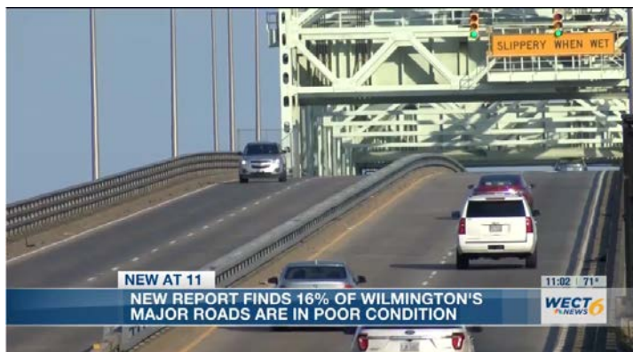
The Cape Fear Memorial Bridge is among bridges that are more than 50-year-old and need to be replaced.
