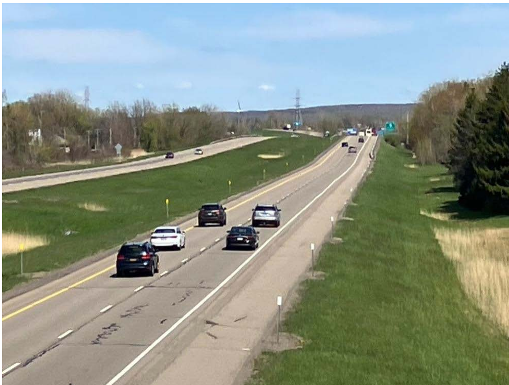
View of Interstate 90 from Brigham Road in Dunkirk. Photo by Greg Larson
