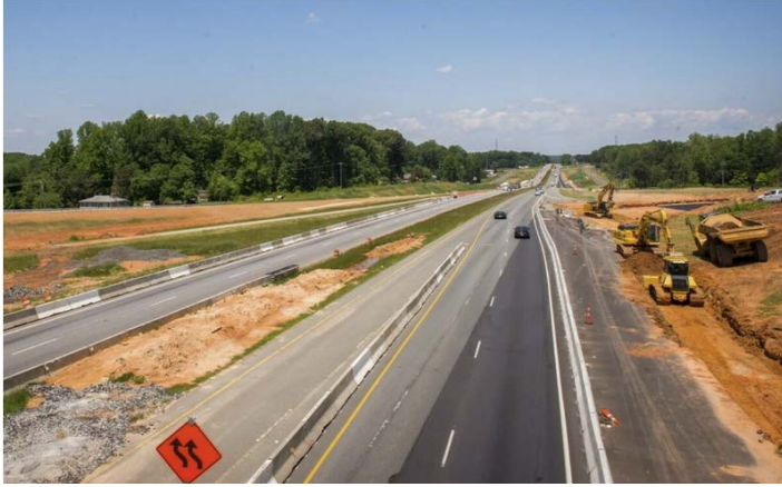
Road Construction. Source: NCDOT
