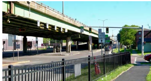
Syracuse's I-81 viaduct is a 1.4-mile elevated stretch that cuts the city in half. On one side is the Pioneer Homes housing project, on the other side is Upstate Medical University. Robert Bell/Rochester Democrat And Chronicle.
