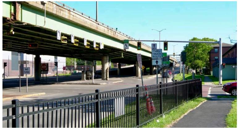
Syracuse's I-81 viaduct is a 1.4-mile elevated stretch that cuts the city in half. On one side is the Pioneer Homes housing project, on the other side is Upstate Medical University. Robert Bell/Rochester Democrat And Chronicle .
