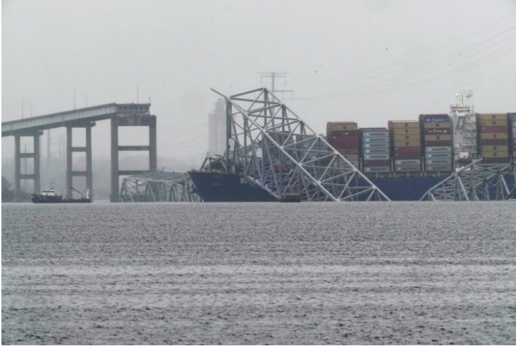
The ruins of the Francis Scott Key Bridge in Baltimore are shown. A study by national transportation research nonprofit TRIP highlights America's ailing and older bridges. (AP Photo)
