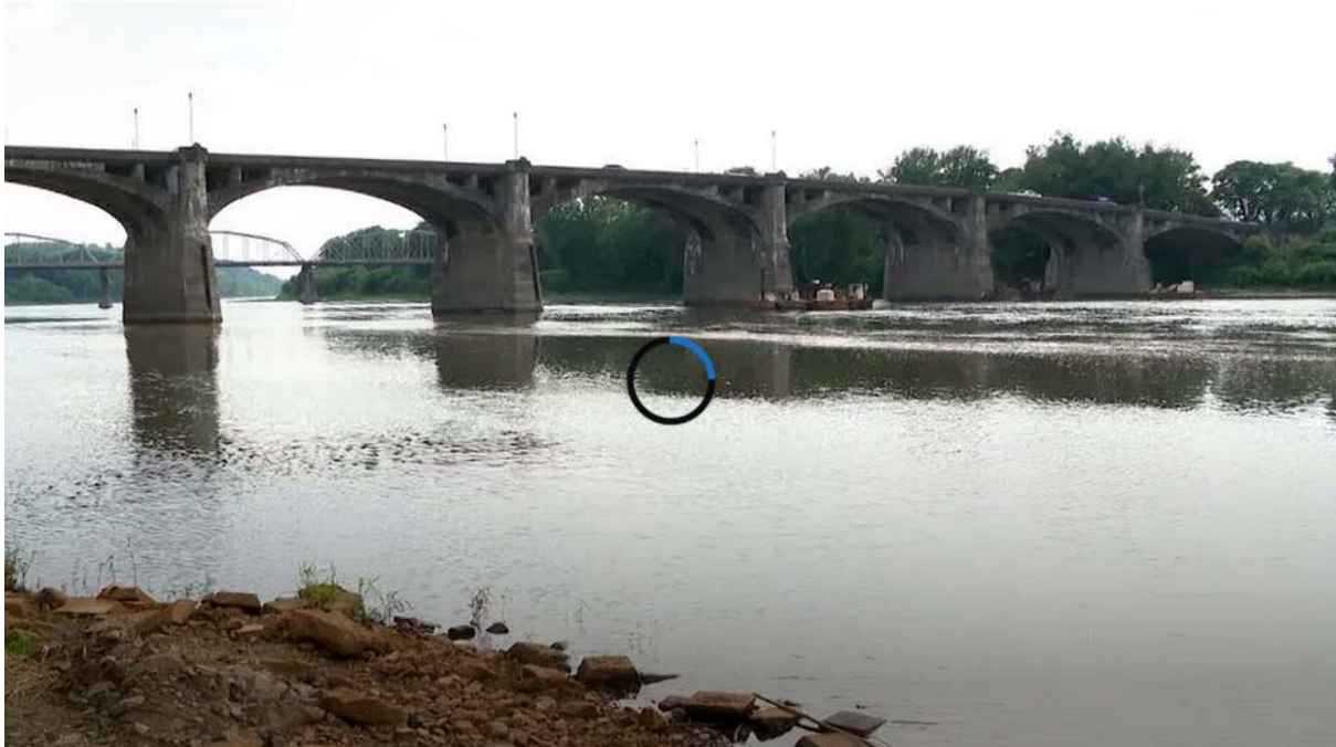
Fort Jenkins Bridge along the Susquehanna River (WOLF)
