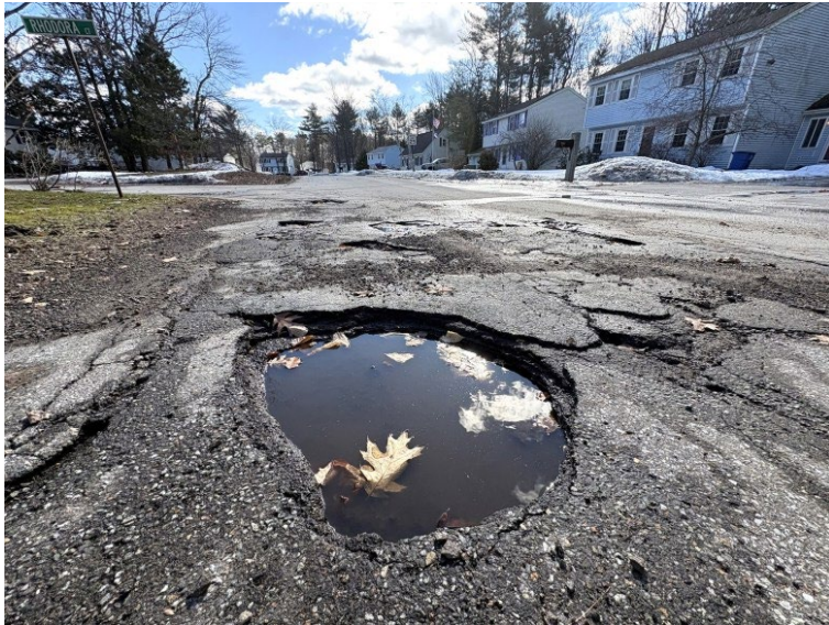
A pothole filled with water on Woodbine Ave in Concord. Credit: GEOFF FORESTER / For the Monitor
