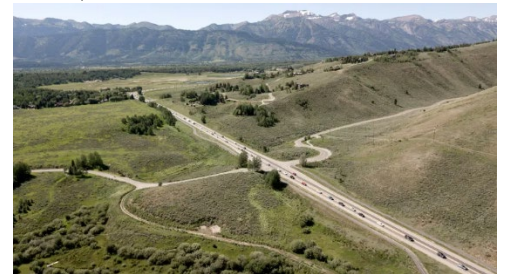
Wyoming Highway 22 connects the town of Jackson to Wilson and climbs Teton Pass, linking the communities of Victor and Driggs, Idaho, to Jackson Hole. A $60 million project would widen a section of the critical commuter artery between Jackson and Wilson. (Ryan Dorgan)
