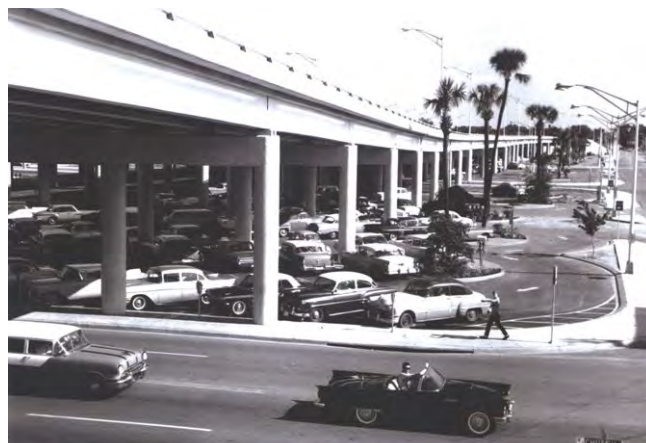
I-4 in Orange County, America to Washington Street in Orlando showing Municipal Parking Area under the large structure on the recently opened project. 7-19-62.
