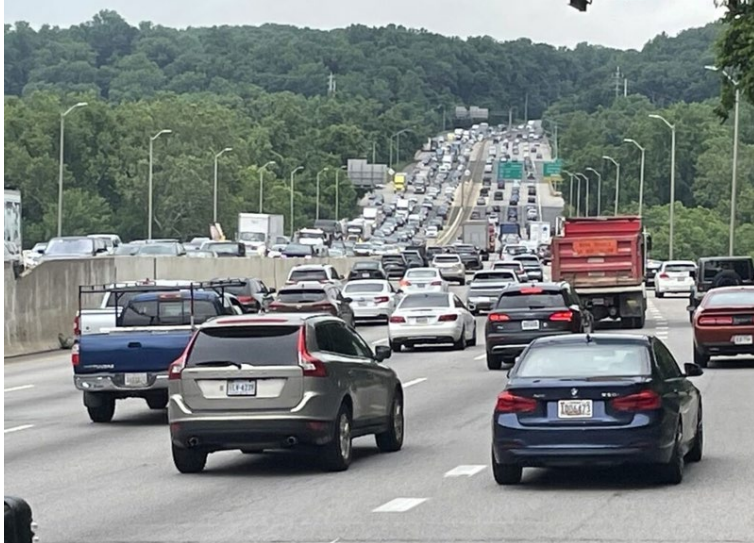
Midday traffic on the American Legion Bridge, which connects Maryland with Virginia, on June 14, 2022. (Photo by Bruce DePuyt/Maryland Matters)
