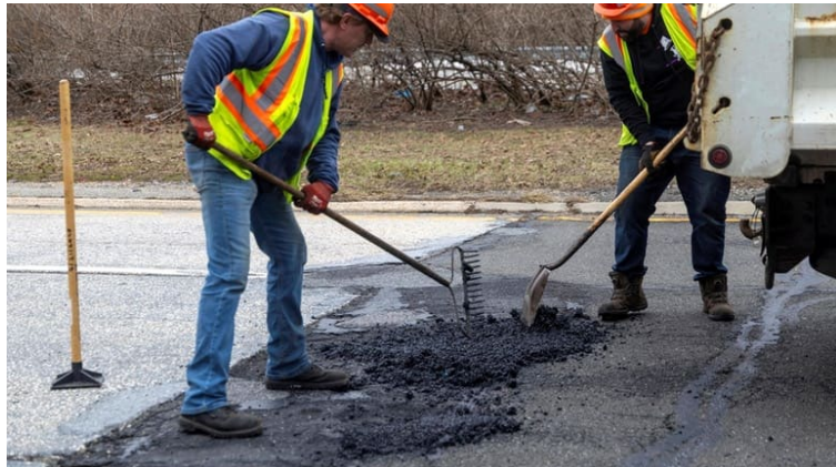
Crews repair a pothole on the northbound Wantagh Parkway in Wantagh in March. Credit: Newsday/Howard Schnapp
